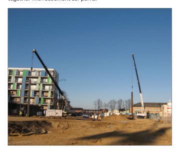
Hill Partnerships appointed Fussey Piling as the sheet piling contractor to design and install a retaining wall around the perimeter of the site, including temporary propping and extraction of the steel sheet piles at a later date.
