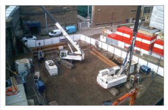
The ground conditions encountered were made ground to a depth of approximately 0.5m, overlaying sand and gravel to approximate 6.5m, overlaying the London clay. Therefore, to ensure that the piles entered the ground smoothly, the ground was pre-augered before installation, using the auger motor mounted on the RTG16T.
