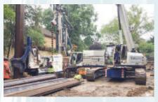
Due to the dense nature of the soils the ground was initially pre-augered with one of our Bauer RTG 16T leader rigs to full pile depth. The 400mm nominal diameter auger loosens the soil without
