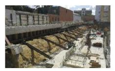
finalised and works were programme to commence on site. This showed, we could pre-auger through the hard soils easily enough without un-necessary wear on the auger equipment and prove drivability of the sheets through this difficult soil band.
