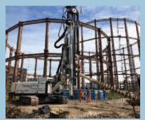
Our smallest project involved the silent and vibration-free driving of just 10 No. 6m sheet piles on a former gas holder site in Bethnal Green. Due to the nature of the ground, the soil had to be first pre-augered with our RTG Leader Rig. Once that operation was completed, we had to mobilise a crane and silent pile press to install the sheets. More time was spent in the 1.5 days on site mobilising and removing the equipment than was spent installing the piles.
